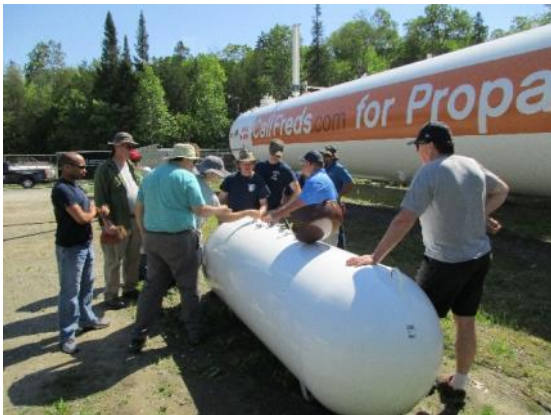
Review of ASME Tank valves and connections
