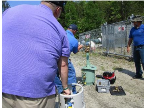
Review of underground dome valves and connections
