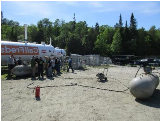
Product transfer w/LPG Compressor
