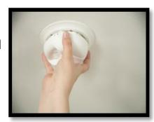
Test smoke alarms at least once a month using the test button. Make sure everyone in the home understands the sound of the smoke alarm and knows how to respond.
